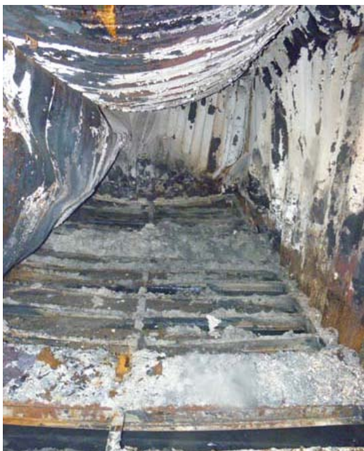
Inside view of MEKP container Photo: Burgoynes
