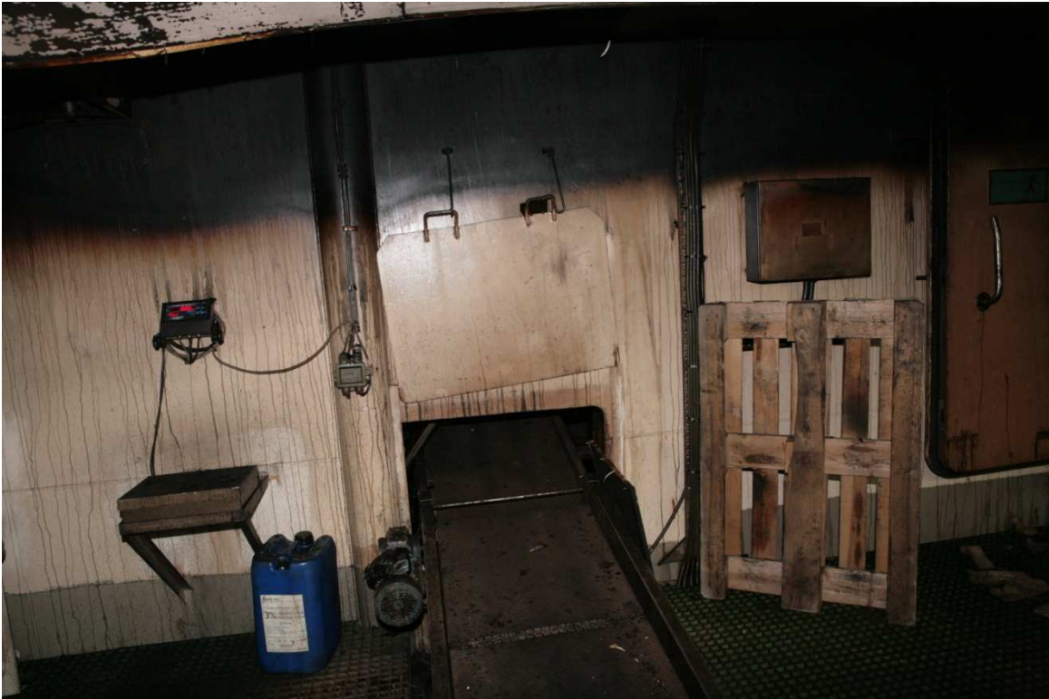
Open sliding hatch viewed from the processing area
