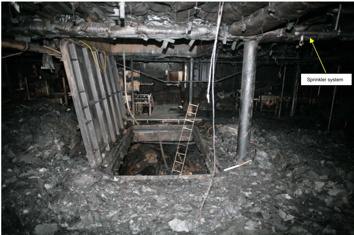
Open hatch on the 2 nd deck, packing room
