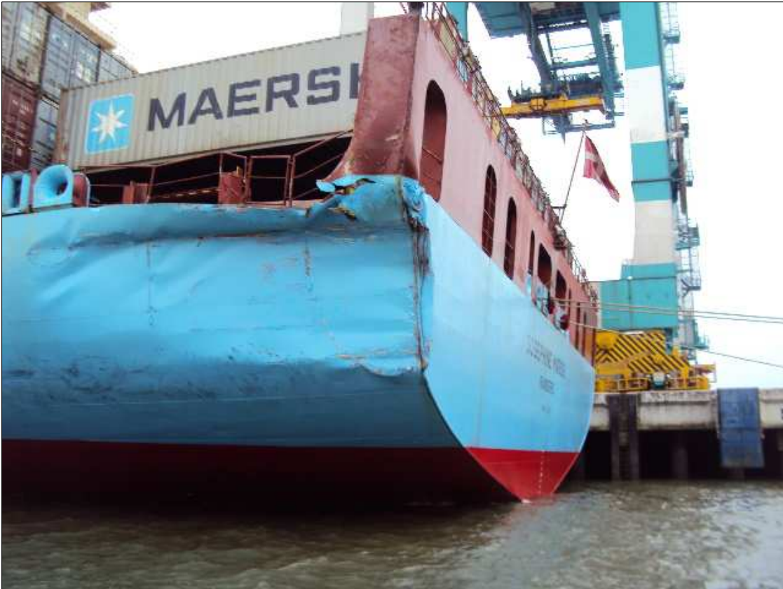
Figure 21: Damage to JOSEPHINE MÆRSK Source: Maersk Line
