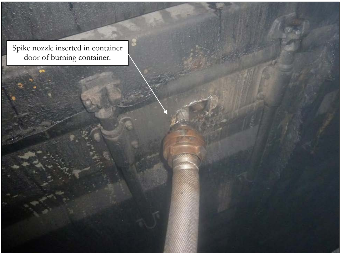
Figure 6: Burning container with spike nozzle inserted.
